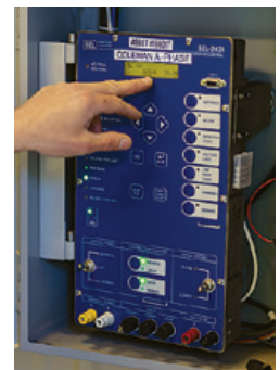
Updated regulator control panels at distribution substations like Coleman in Grand Forks will help Minnkota’s control center better monitor and respond to fluctuations in voltage.
