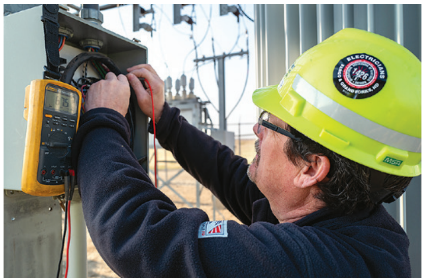
Minnkota technical maintenance technician Perry Flaten checks for proper voltages in the CT/PT box at the Coleman substation.
