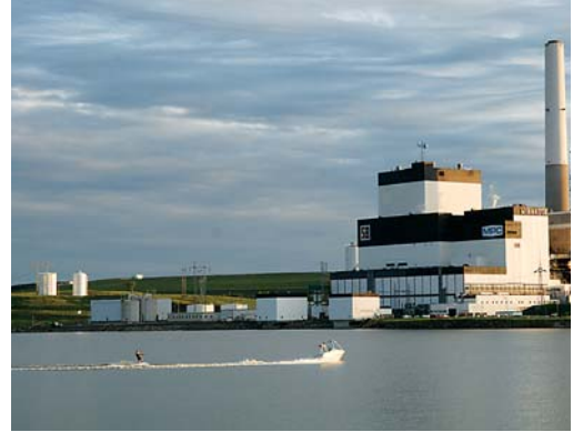
The warm water discharged from the plant means Nelson Lake rarely freezes, making it unique among North Dakota's lakes.
