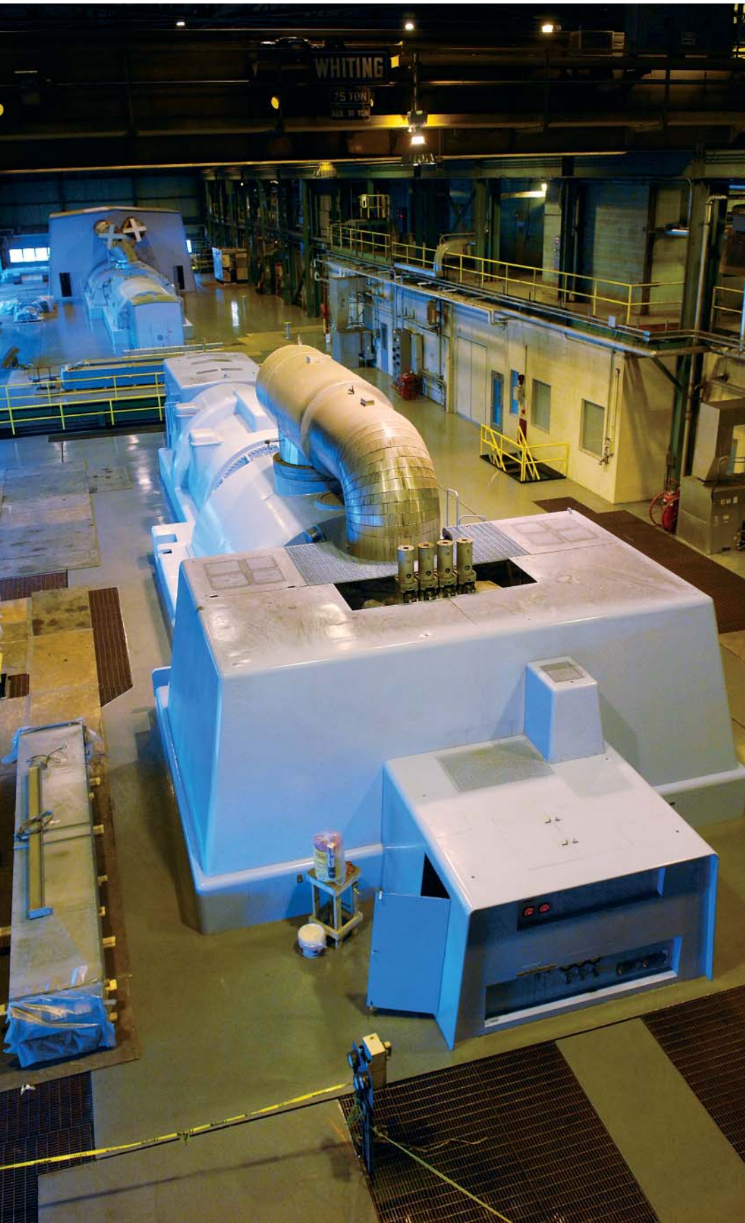
Each of the two units at the Young Station has a turbine generator. Inside each generator, a huge spinning magnet surrounded by coils of copper wire creates a magnetic field which, in turn, creates a flow of electricity.
