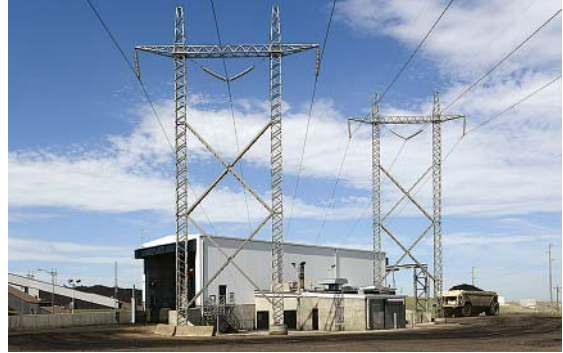
Lignite coal is transported in as large as 240-ton haulers from the nearby Center Mine to the plant site, where it is dumped into underground hoppers and moved along feeder chains to the primary crusher.
