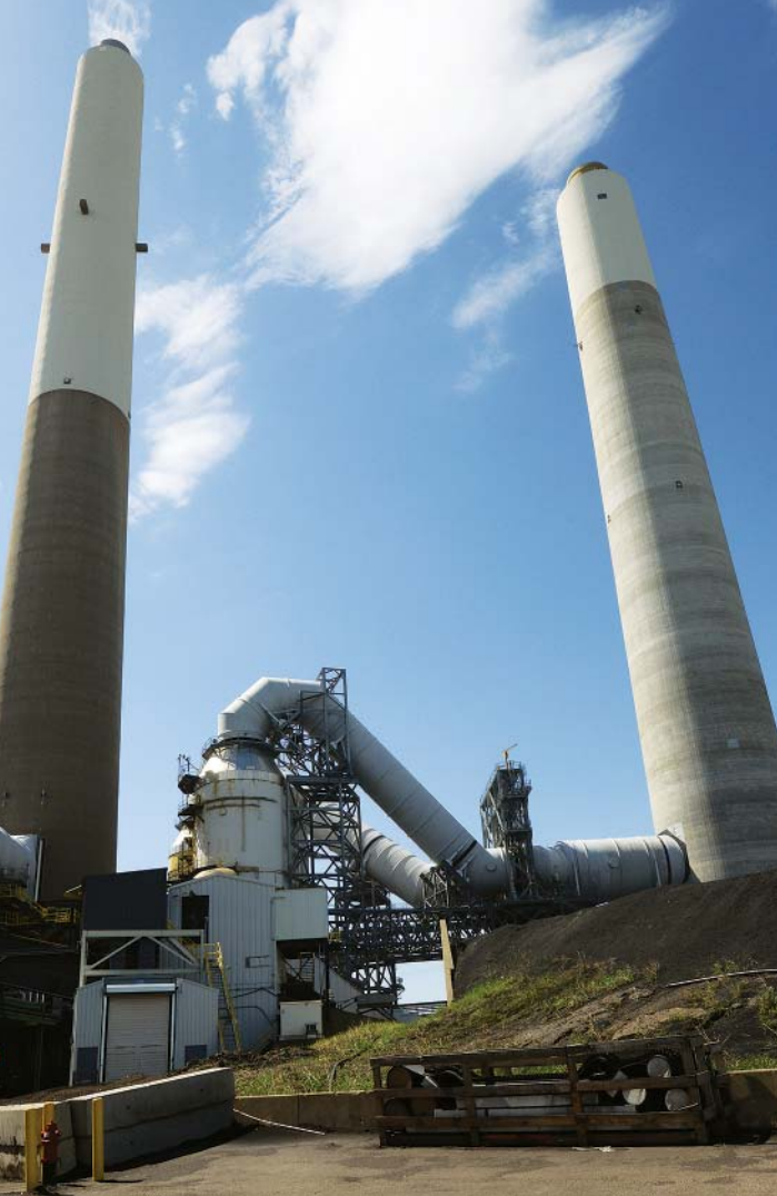
The new Young 2 chimney (right) was constructed to handle the wet flue gas produced by the unit's scrubber. The old Young 2 chimney was then modified for Young 1 to use.
