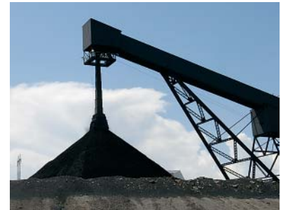
After the coal is crushed, it is conveyed to storage piles for use at the Young Station.
