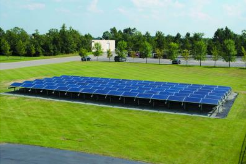
Beltrami Electric Cooperative's 80 kW Northern Solar Community Solar Garden Bemidji, MN
