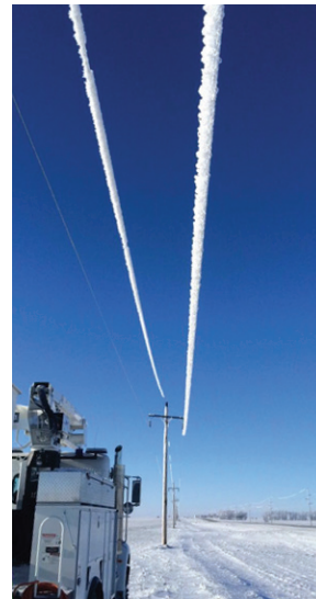
The northeast region of North Dakota is especially prone to ice storms, so sights like this are common for Langdon-area line crews. CREC's Marty Tetraault says they have even buried some lines to avoid the recurring issue. Photo courtesy of Ron Hanson.
