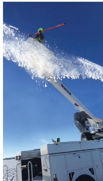
Sometimes clearing the lines just takes some muscle, with crews using insulated hot sticks to smash the ice. Photo courtesy of Ron Hanson.
