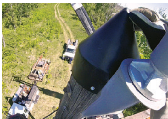
A poletop helmet is installed on top of the structure to prevent birds from nesting and perching on the structure.
