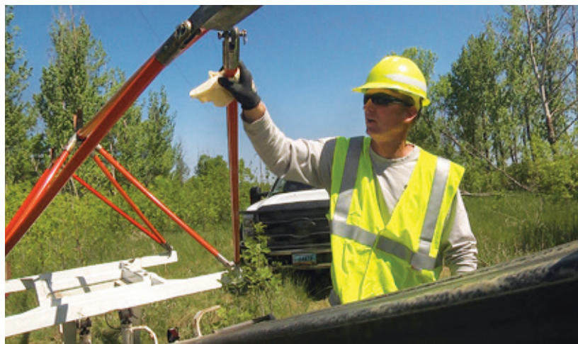
Kelly Hebl, heavy crew foreman, cleans the insulated jib that raises the energized wires overhead so work can be completed safely.
