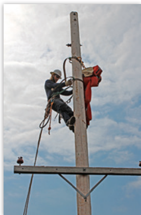
Apprentice Lineman Ben Pahlen performing a pole top rescue for a MREA safety meeting.
