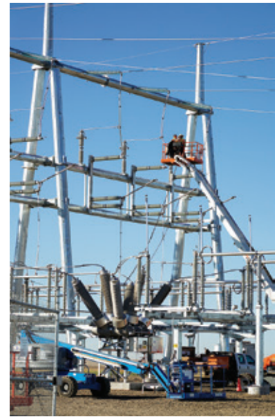
Minnkota crews work on the Roughrider substation, which connects the Oliver III wind farm to the electric grid.
