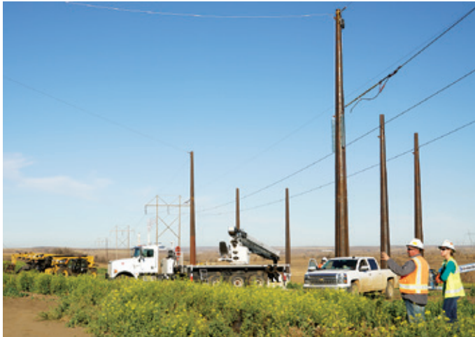
Crews stand near a newly constructed stretch of 230-kV line that transmits power from the wind farm.
