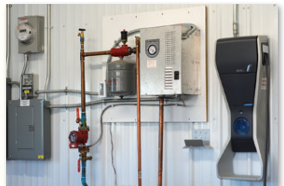
The first Level 2 electric vehicle charging station on Minnkota's demand response program was installed late last year. (Above) A 240-volt charging station (seen on far right) can fully charge a vehicle's battery in 2 to 4 hours.
