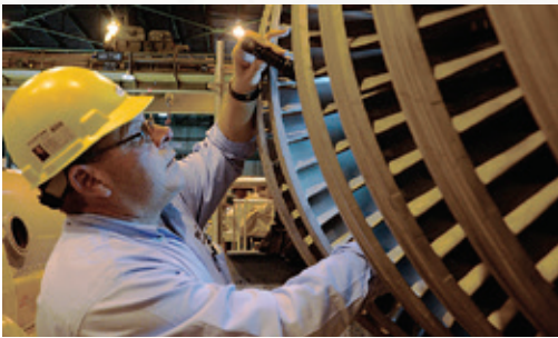
Paul Koedam, maintenance supervisor, inspects the HP-IP turbine blades during the Unit 2 major outage.
