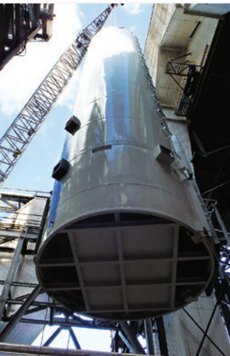
Using its 315-foot boom, a crane positions the new powdered-activated carbon silo onto its foundation.
