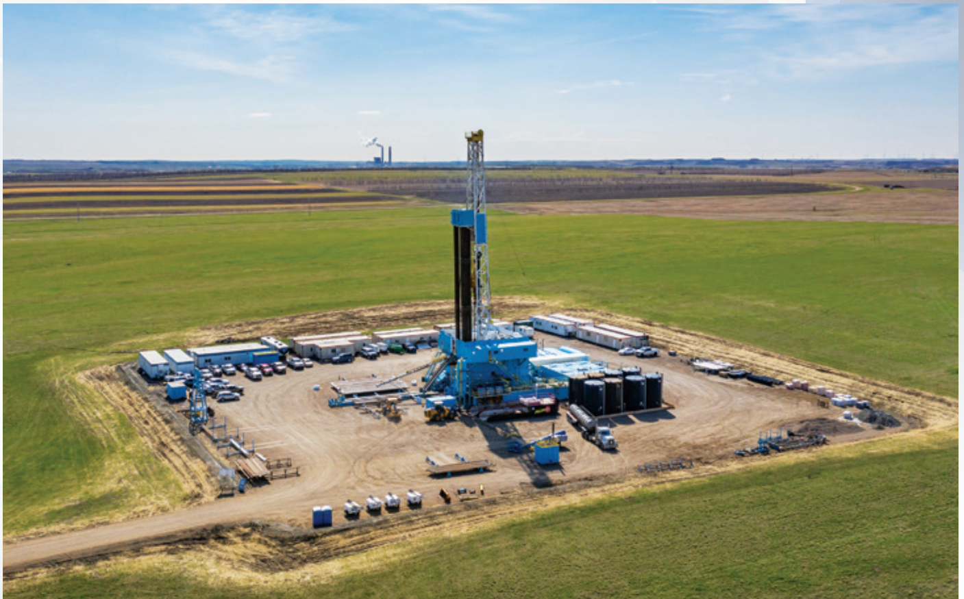
Small water injection tests were performed this winter at a test well site south of Center, N.D. The results showed the local formations would safely accept CO 2 at the rate and volume needed for Project Tundra. (Submitted photo)
